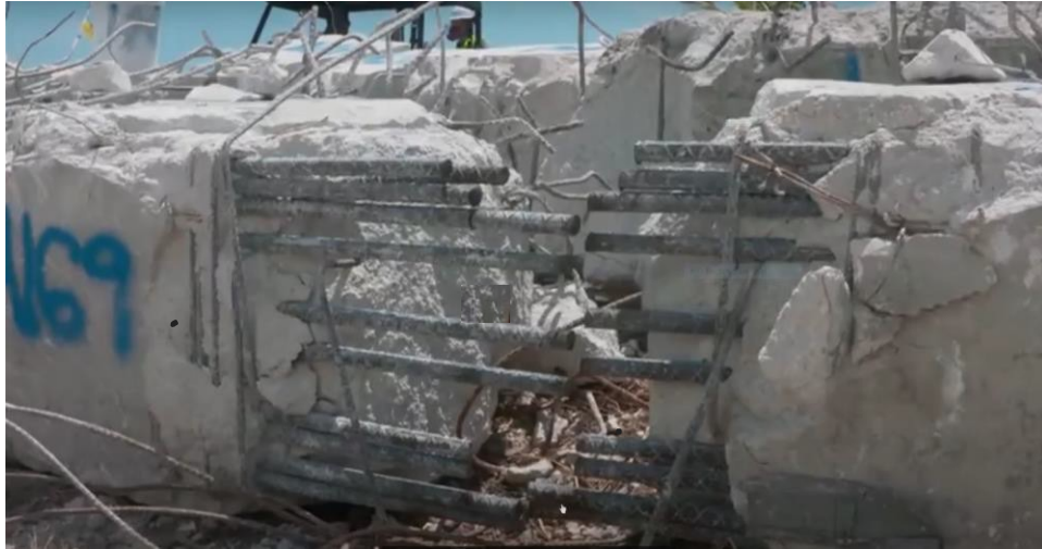
Proximity of reinforcing steel in building and garage columns
