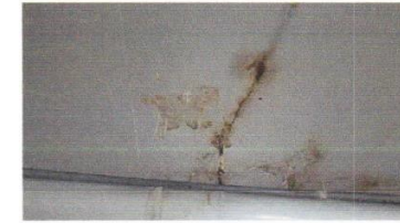
Figure K2: More previously installed failed injection repairs with leaching forming
