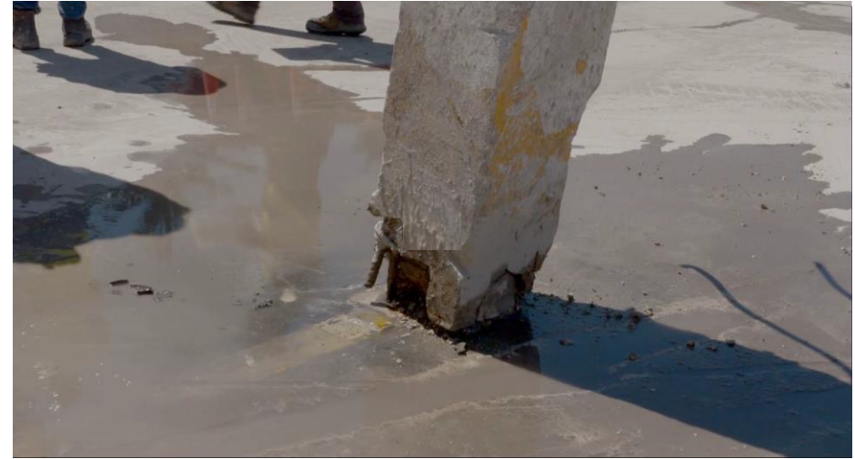
Corrosion of columns at garage slab and foundation
