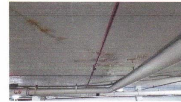
Figure K2: More previously installed failed injection repairs with leaching forming
