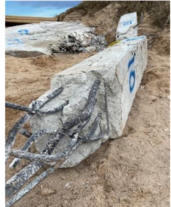
Column to beam connections
