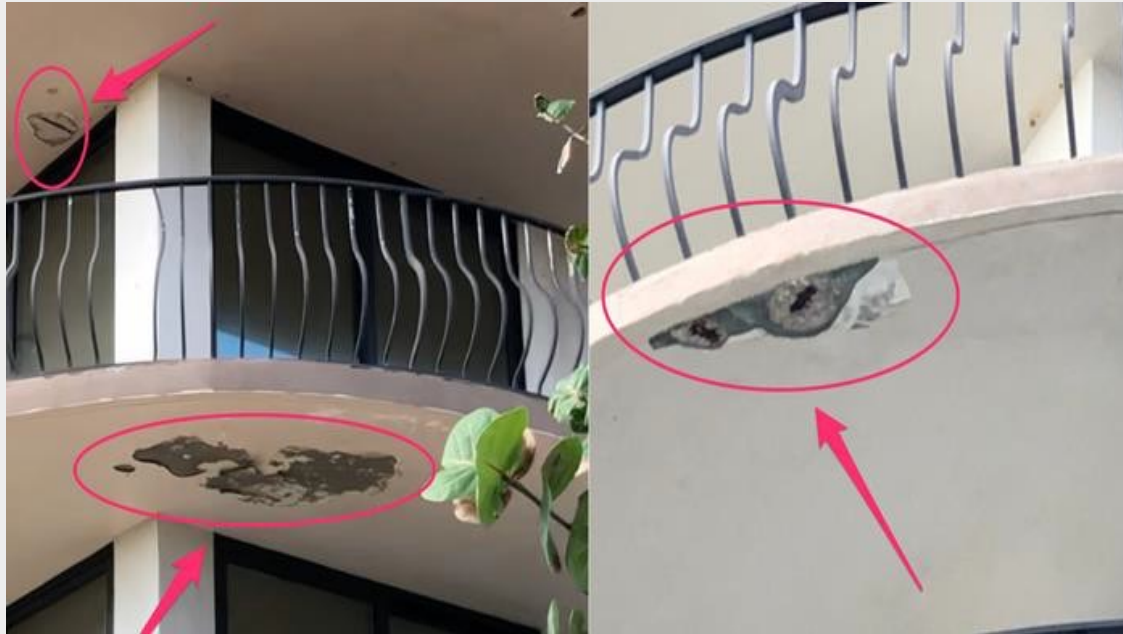
Spalling concrete at balconies
