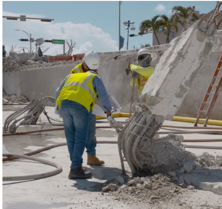
Column to foundation connections
