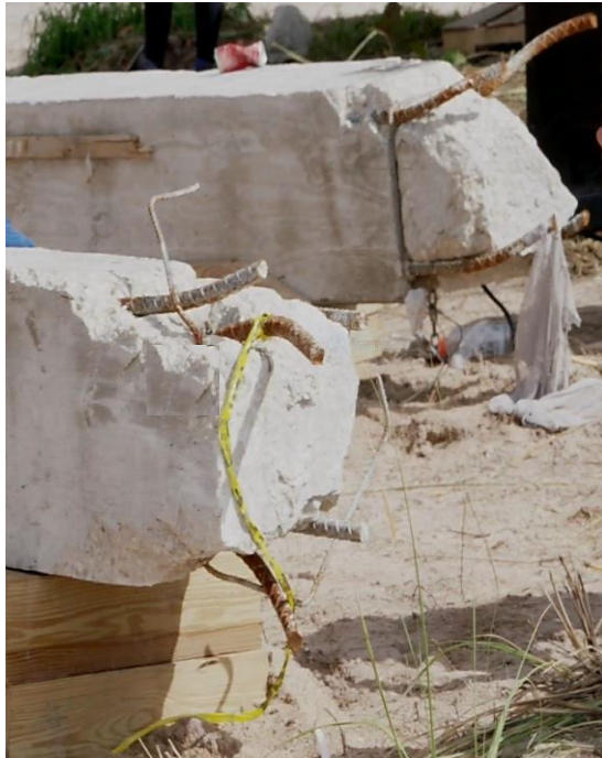
Amount of reinforcing steel in columns
